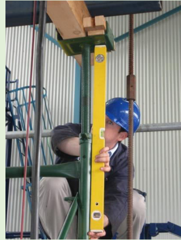
PHOTO B: Measuring effect of load application
